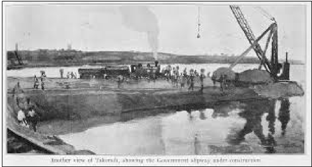
Figure 4.57 Construction of Takoradi harbour During 1920s
