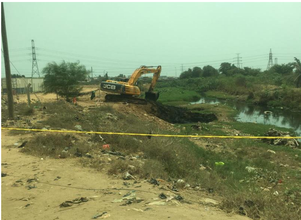
Plate 5.2-1 Dredging of Lower Reaches of Chemu Lagoon
