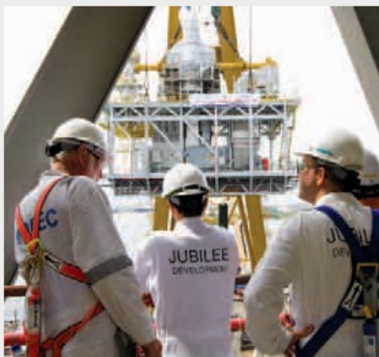
Process module installation, FPSO Singapore
