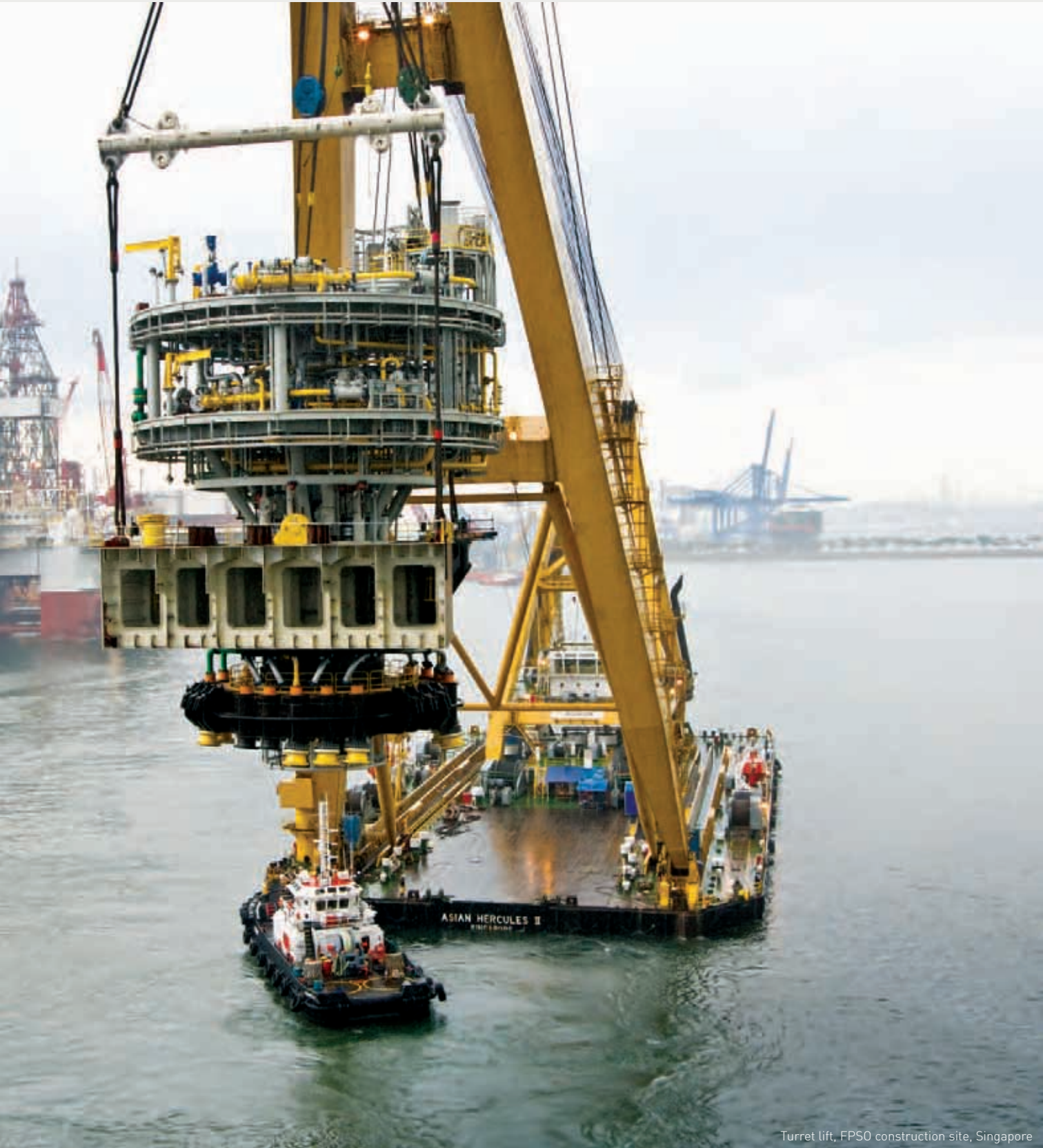
Turret lift, FPSO construction site, Singapore
