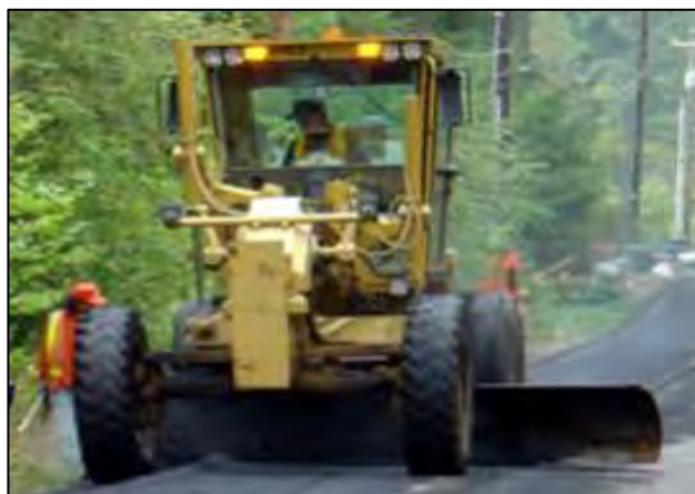
Figure A-8 Typical road spreading operation
