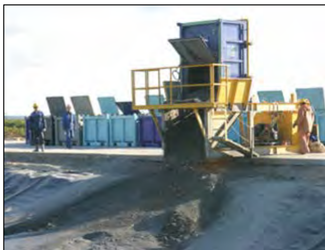
Figure A-9 Typical landfill operation
