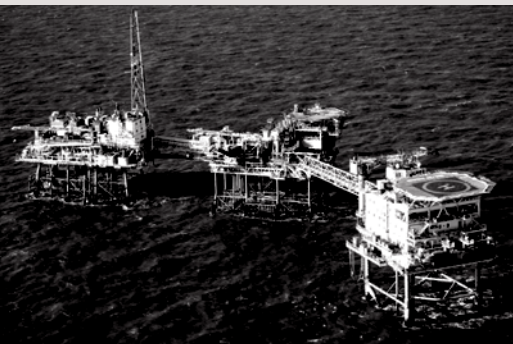
The central processing complex on the Hewett field, in the UK's Southern North Sea.
