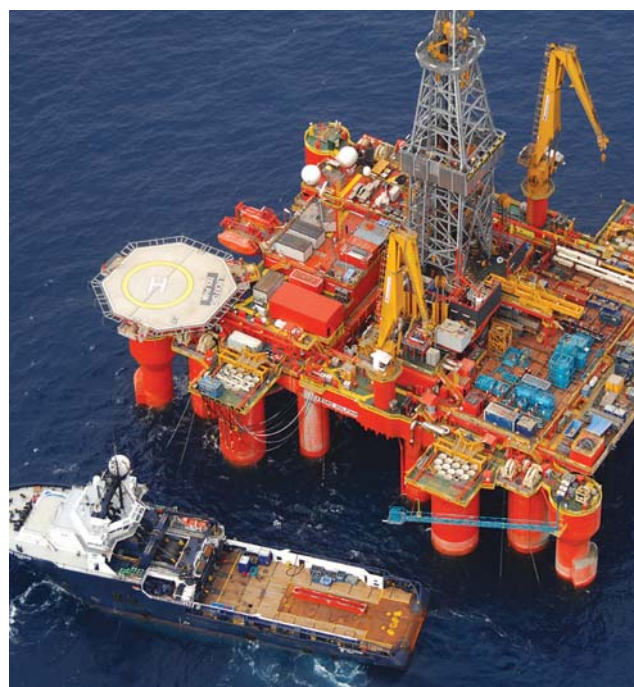
Blackford Dolphin rig drilling Hyedua-2 appraisal well offshore Ghana.
