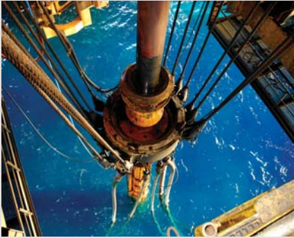
Drilling riser on Eirik Raude rig, offshore Ghana.
