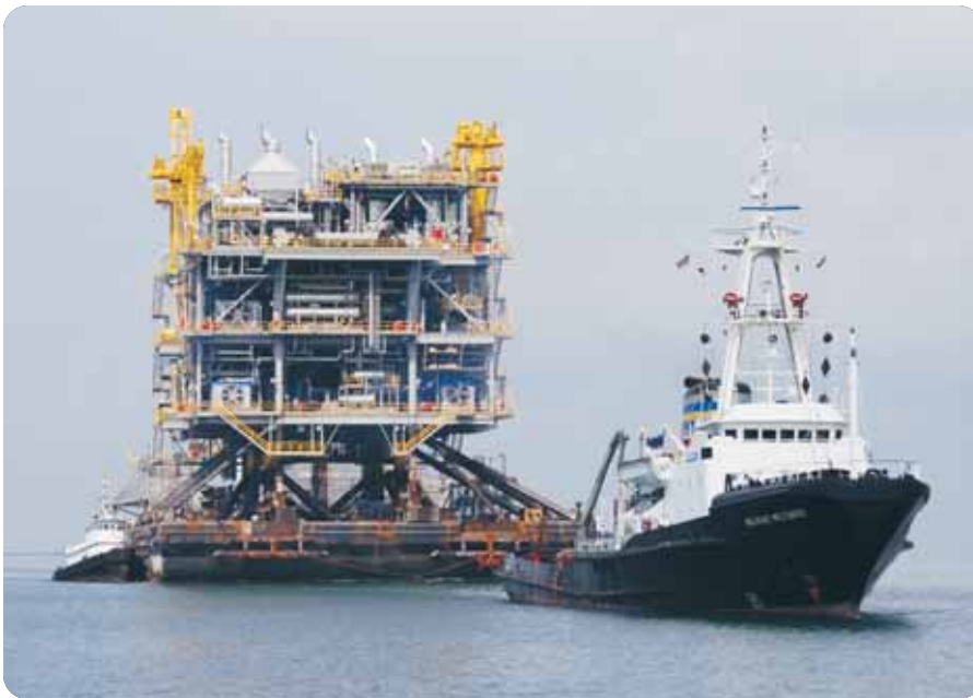
The Central Processing Facility in transit to the Okume Complex in Equatorial Guinea. First production from the field commenced in December 2006.
